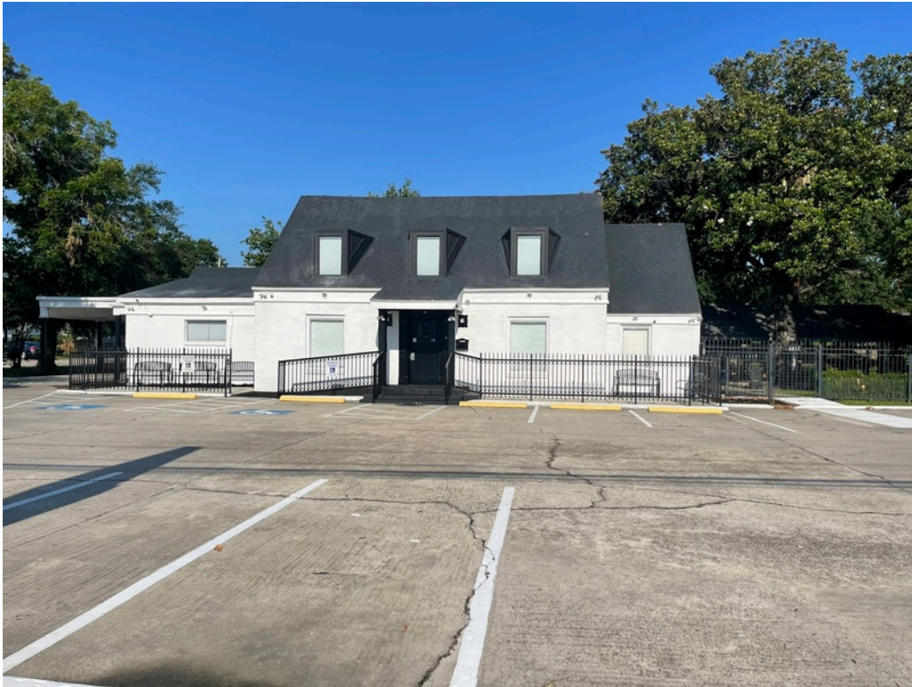
15. East adjoining property (VJW Clothiers)
