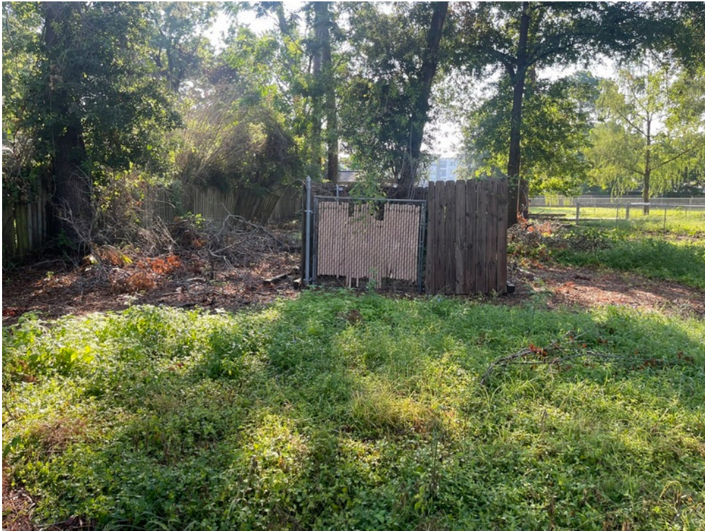
5. Dumpster enclosure in northwest portion of subject property
