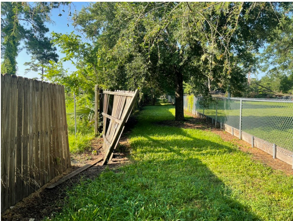
10. View south along east property boundary
