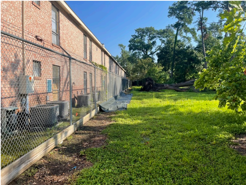
12. View north along west property boundary
