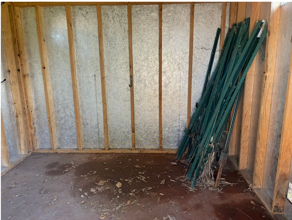
4. Interior of onsite storage shed
